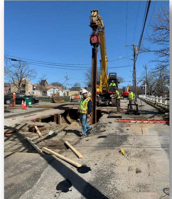
Sewer installation continues within Main Street, Hyannis
